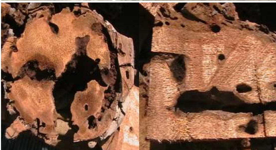
Fig.9. Damages by Oryctes spp., holes in trunk (Source: M. Zaidan Khalaf)
