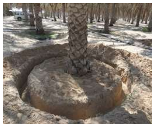
Sub-surface irrigation system
